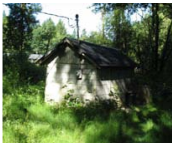
South Keyport Heights Pumphouse
