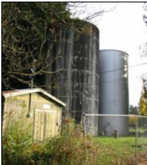
Storage tanks that belong to the Delta Water Association
