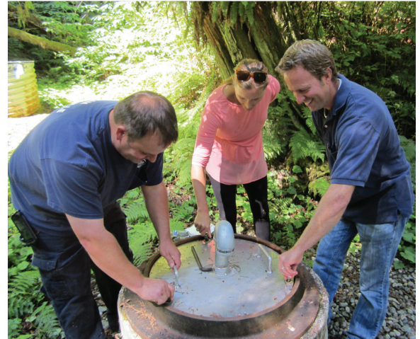
Staff at Marysville Utilities, (from left) Billy Gilbert, Kari Chennault, and Brad Zahnow, open and inspect a spring collector to ensure there are no sanitary defects.
